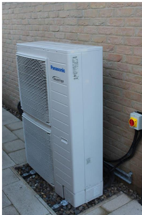
Fig. 5.4 – Typical Air Source Heat Pump Installation
